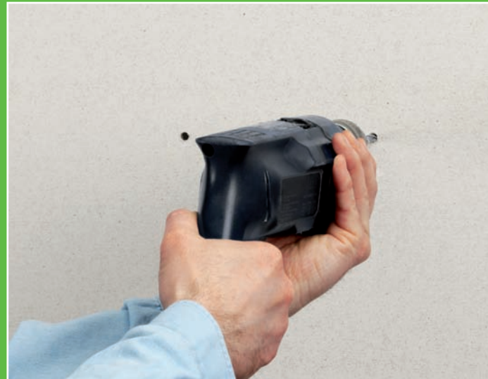
2. DRILL (with standard 6-mm bit)
