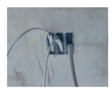
▲ Trouble-free transition of cables out of the ceiling into lightweight construction walls to be created underneath.
